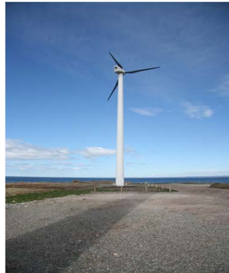
Turbine 1 in the Ramea Wind Farm with wooden stakes in foreground marking some of the distance sectors around the installation that are used in the estimates of observed bird distances from turbines and in carcass searches and experiments. (photo by: W. A. Montevecchi)
